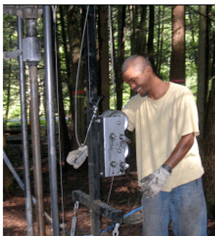
Figure 2a) Terry Daniels (PSU undergrad) drills wells with the Portadrill Mini.
