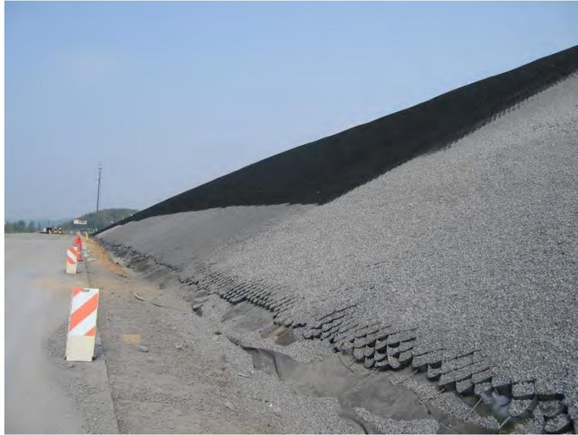
**Figure 4. GeoWeb covering of the Buttress/Bifurcation Fill**
