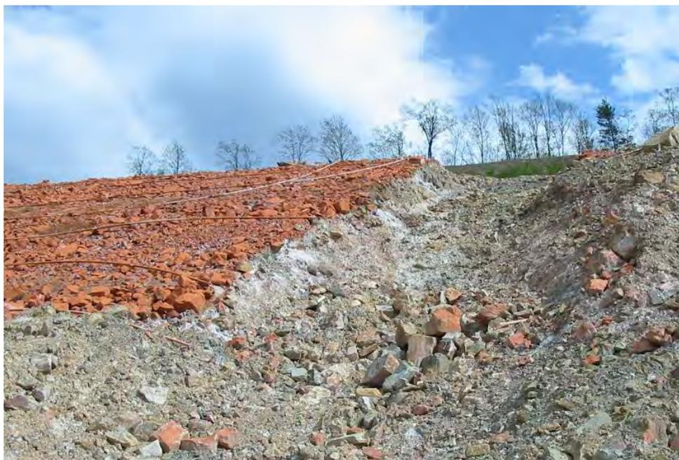
**Figure 12.** View of Bauxsol™ treated area at Skytop. Orange colored Bauxsol™ coated rubble remains on left side of image. Also shown are sprinkler pipes used to distribute the Bauxsol™ slurry over the surface. A trench dug through the rubble is on the right side and foreground in this photograph. As shown here, Bauxsol™ penetration depths into rubble were limited to less than 2 feet.
