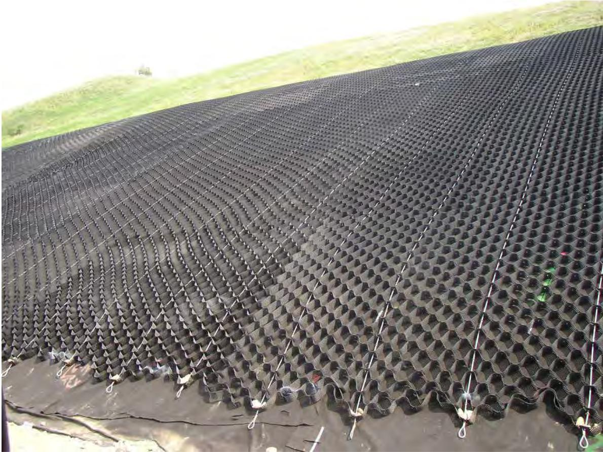
**Figure 9.** *GeoWeb textile held in place by stainless steel cables. The fill/cover of limestone aggregate has yet to be added.*
