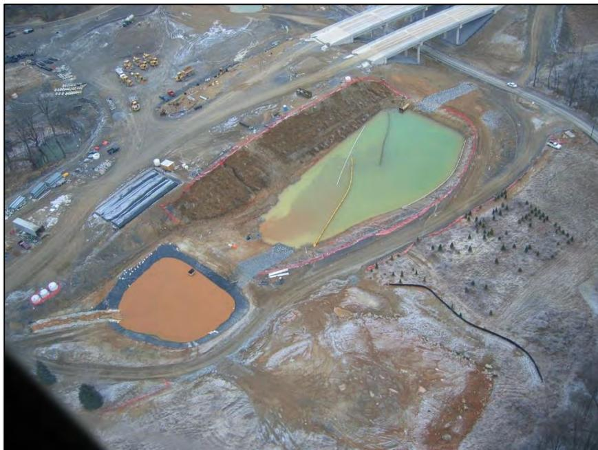
**Figure 7. Photo of temporary surface water-treatment ponds**
