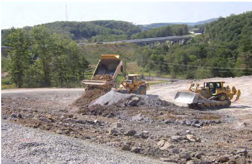
**Figure 5. Initial construction of the Engineered Rock Placement Area.**
