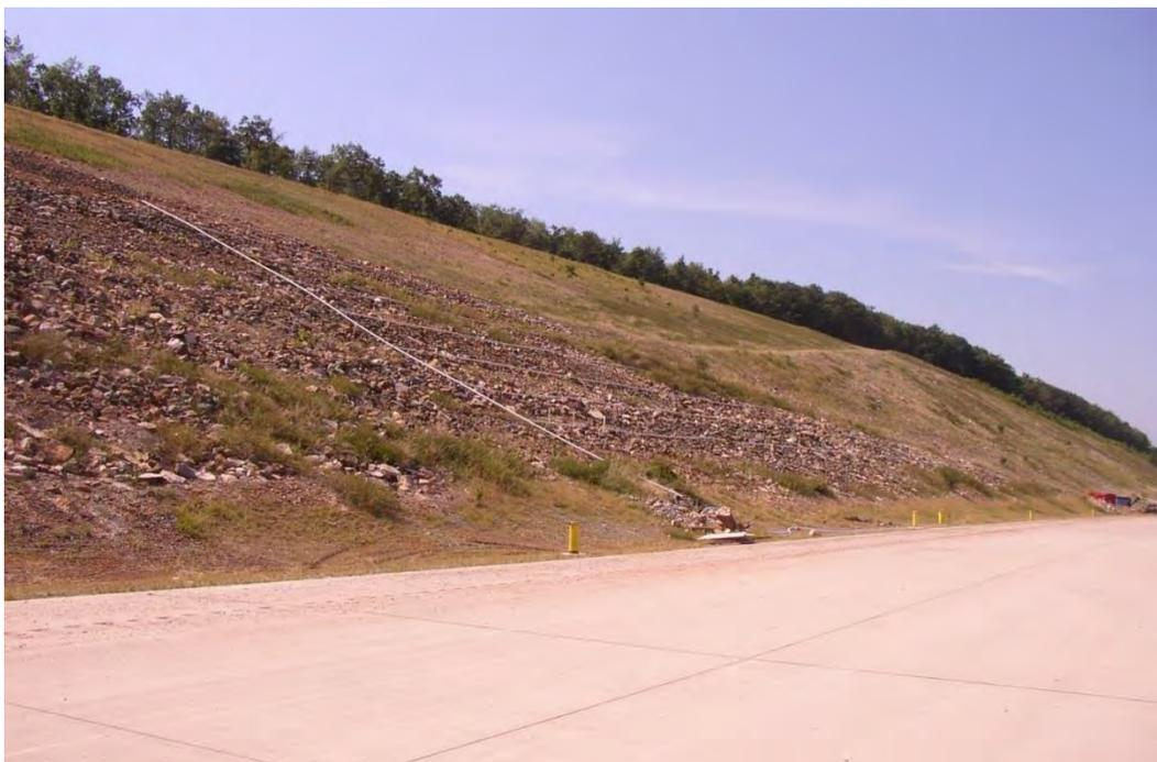
**Figure 4. Test site on the large buttress for spray application of Bauxsol™ across drainage divide in Section C-12.**
