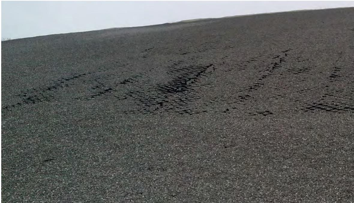
**Figure 10.** *Slumping of limestone aggregate on GeoWeb remediation system, exposing its textile webbing.*
