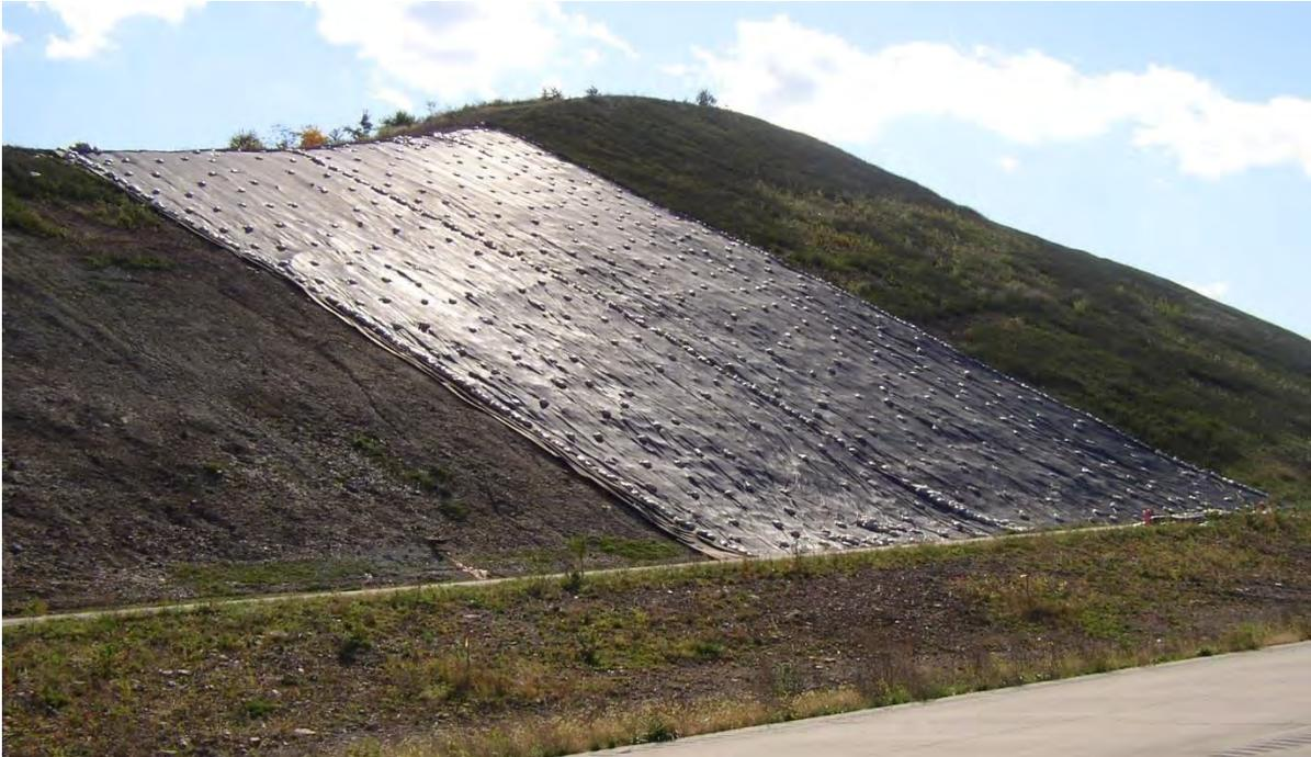
**Figure 23. Small Cut Face with temporary PVC cover over transgressive vein system 300 feet wide.**
