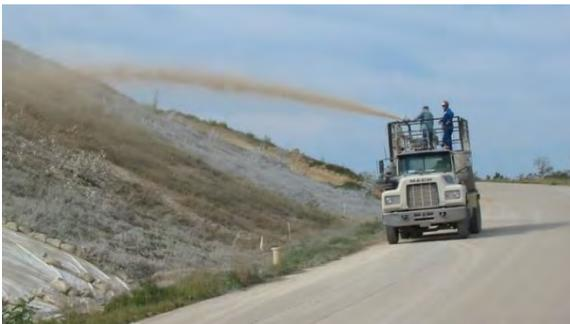
**Figure 15.** Spraying of a slurry at Skytop.
