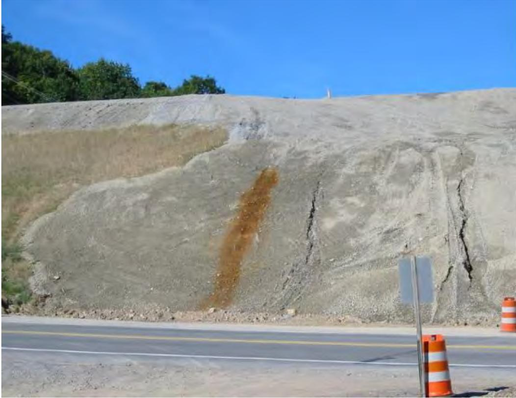
**Figure 3. A point source acid break-out in a powdered limestone-hosted fill on the S.R. 3042 embankment. Reactions were inhibited by armoring of gypsum.**
