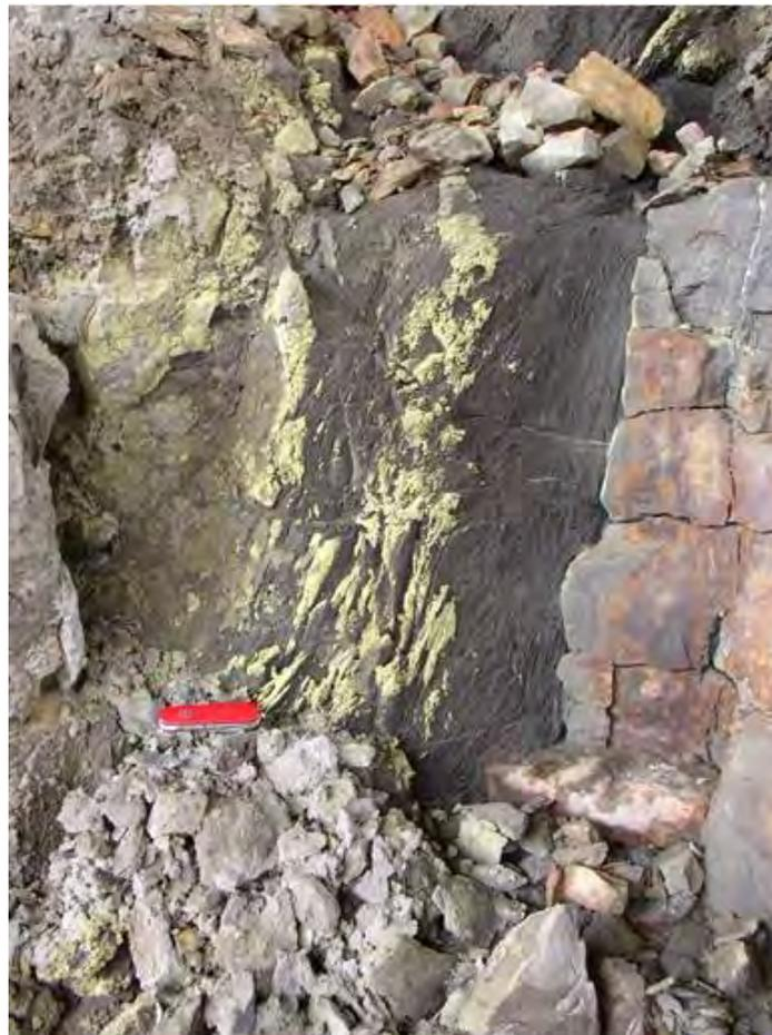
**Figure 20. Copiapite (yellow mineral) in a bridge footing.**
