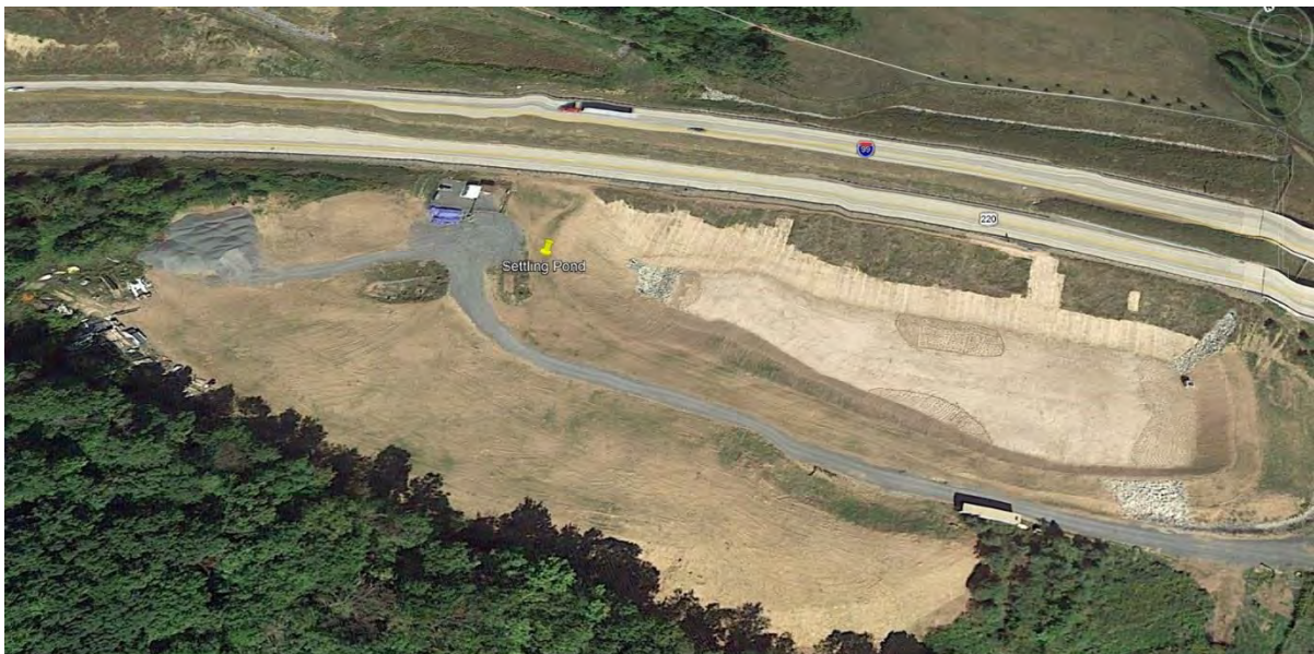
Figure E5-2. Aerial view of settling pond stop.
