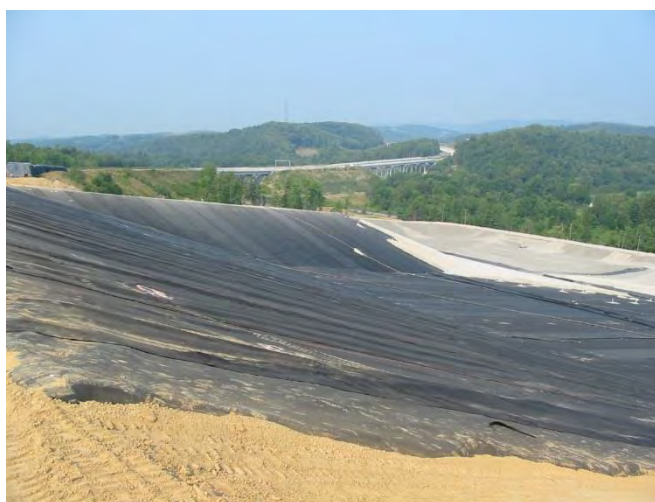
Figure E6-6. Engineered Rock Placement Area (ERPA)
