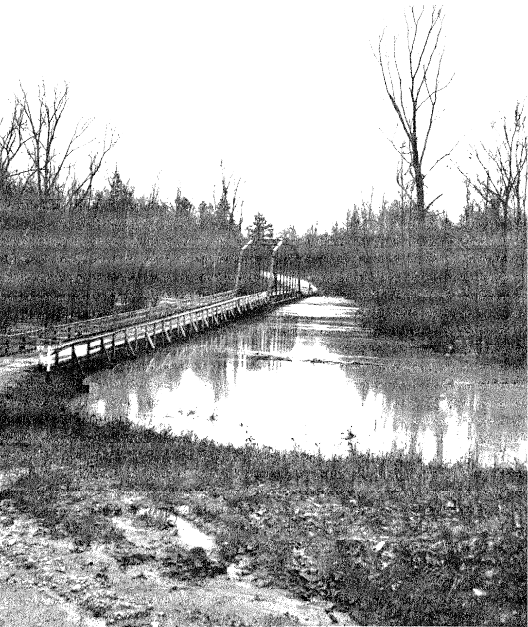
Figure 12.—Bridges in the Piedmont have to span the flood plain as well as the river.
