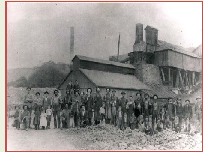
Coal burning at the Greenwood Furnace produced 4 tons of iron per day (1834-1904)
